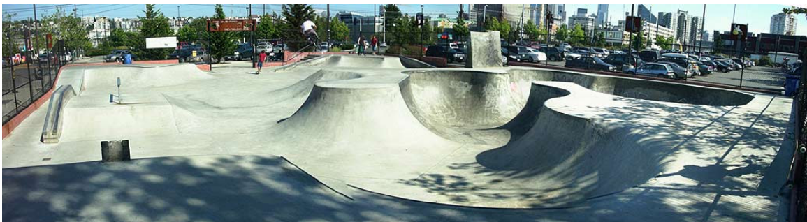
Figure 27: Seattle Center Skatepark. Photo courtesy Dan Hughes
