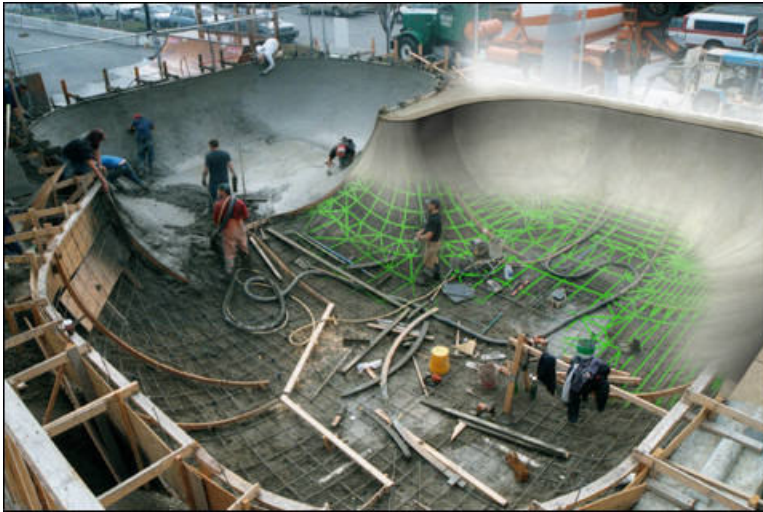
Figure 3: Ballard Bowl during construction. Digitally enhanced photo courtesy Grindline.
